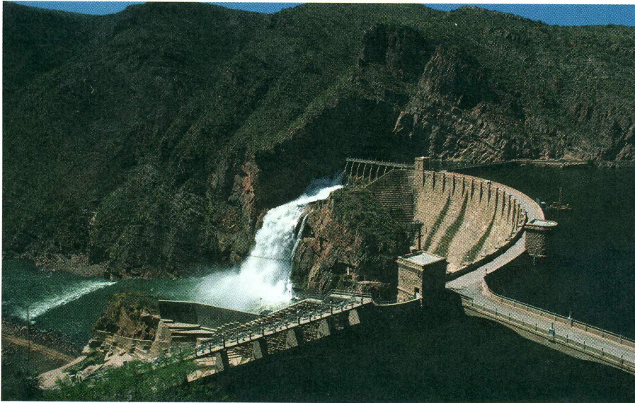
FIGURE 2.12 Potential and kinetic energy. The water stored behind this dam has potential energy. The potential energy is converted into kinetic energy as the water flows through the gates.
